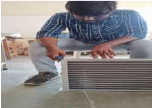
fig.5: Releasing nitrogen gas from the tubes for the inspection
