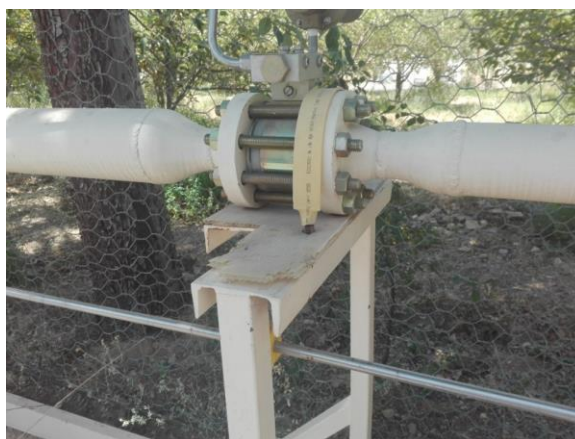
Figure 2. Metal support of the station under study
