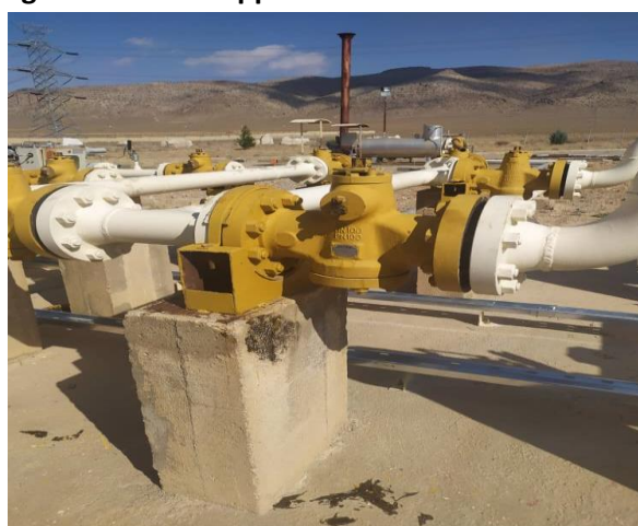
Figure 3. Concrete support of the station under study
