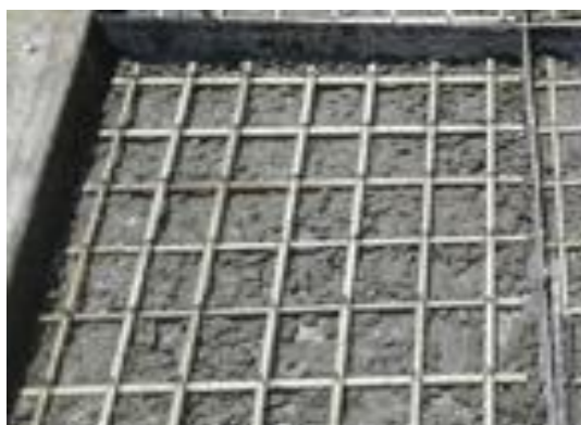
GS1 Slab Bottom mat
