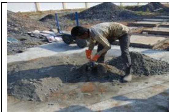
Dry mixing of ingredients
